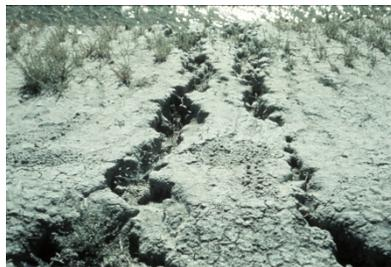
**Figure 4-1 An example of eroded dike slopes.**
