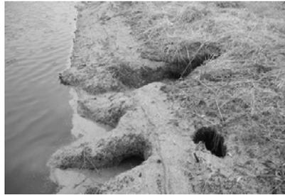
**Figure 4.2 Evidence of burrowing at the edge of a treatment pond (Mayo et al., 2010).**
